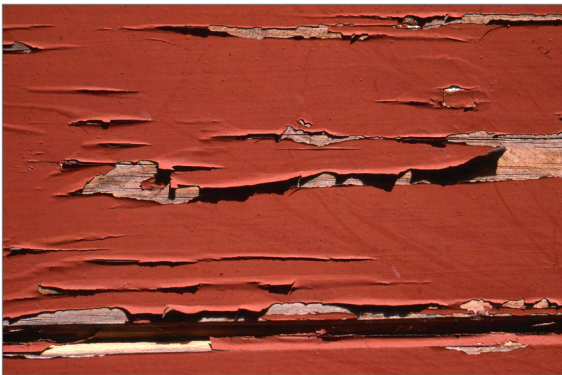
Asbestos and lead paint are well-documented hazards to human health. Courtesy: Brasil2/Getty Images (top); westphalia/Getty Images (bottom)
